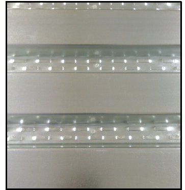
Mill Fresh Steel Deck
